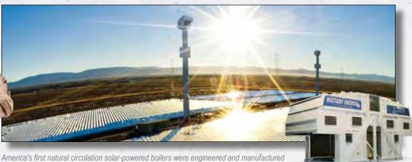
by Victory Energy. The boilers have consistently produced super-heated steam with an average operating temperature of 800°F at a pressure of 900 PSI. Each receiver produces approximately 2.5 MW of power to the grid.
