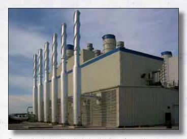
Free standing single wall stacks designed and manufactured by Victory Energy.
