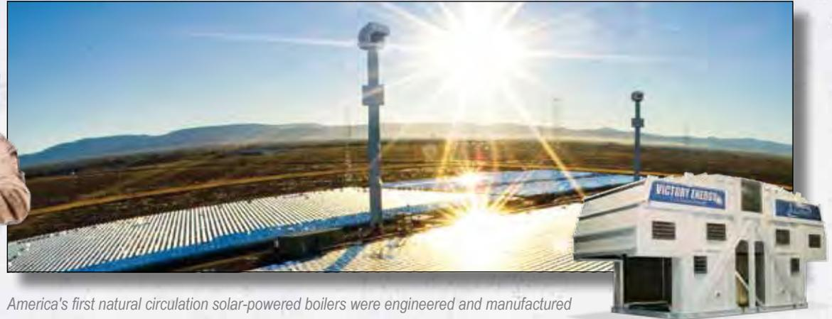
America's first natural circulation solar-powered boilers were engineered and manufactured by Victory Energy. The boilers have consistently produced super-heated steam with an average operating temperature of 800°F at a pressure of 900 PSI. Each receiver produces approximately 2.5 MW of power to the grid.
