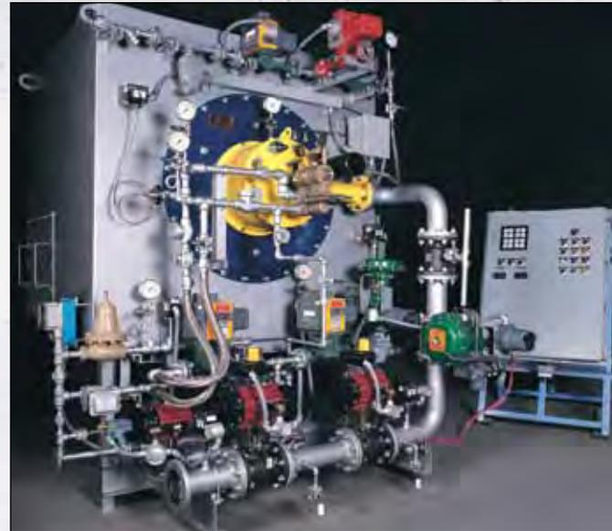
Low or Ultra-low NO<sub>x</sub> burners are supplied for the Voyager and Discovery packaged watertube boilers.
