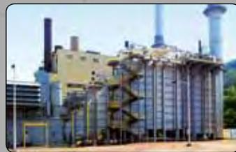
Modular designed, field-erected utility combined cycle HRSG.
