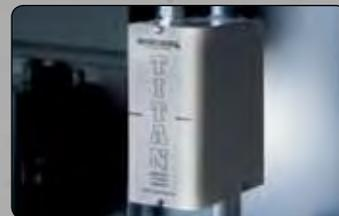
The auxiliary low water cut-out assembly provides an extra measure of safety for the critical drum water level condition.
