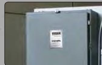
The relay panel assembly provides the relay logic power for the water column and ALWCO probes.
