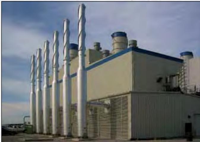
Free standing single wall stacks designed and manufactured by Victory Energy.
