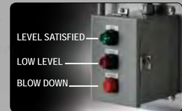
The by-pass station is used for blowdown, a routine preventive maintenance process.
